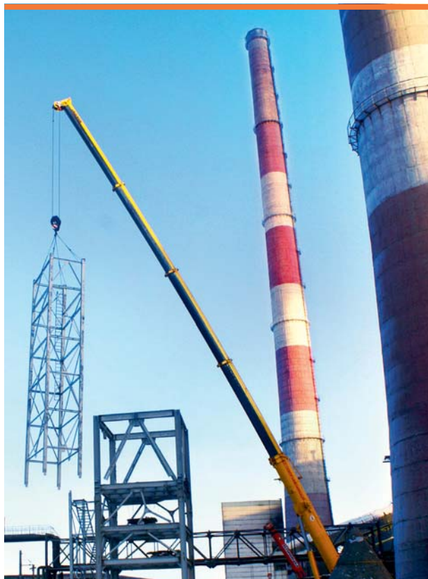
Construction and installation works. Troitskaya GRES
