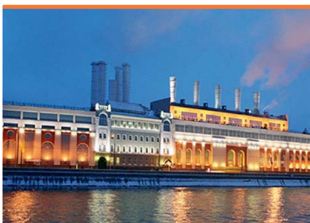
Hydro Power Plant GES-1, Mosenergo.
