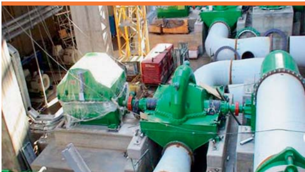
Horizontal and vertical centrifugal single-stage with a scroll case pumps
