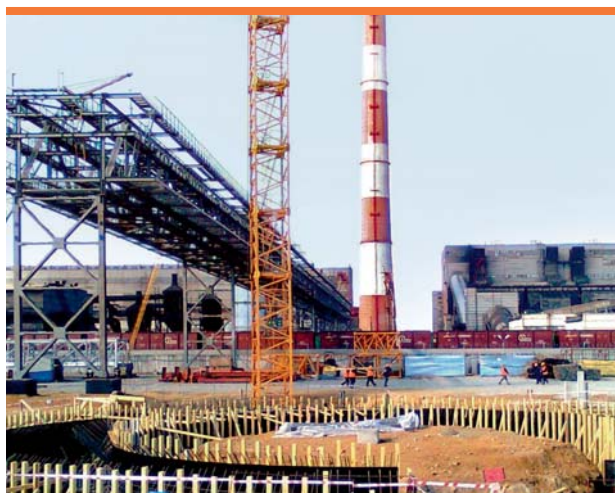
Construction and installation works. Reftinskaya GRES
