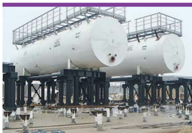
Tank equipment installation. Urnskoye field
