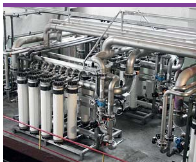
JSC LUKOIL-Komi: Formation waters purification with capacity 700 m 3 /h, \text{æ} \leq 1.0 \mu\text{S}
