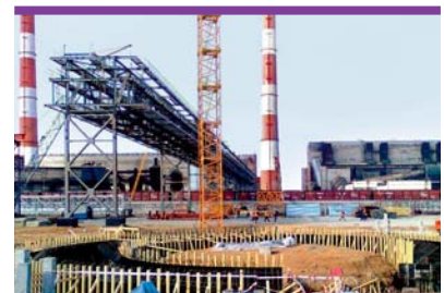
Construction and installation works. Reftinskaya GRES
