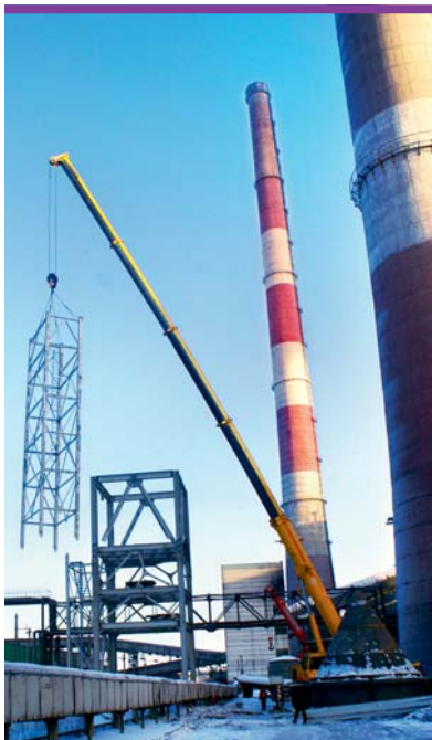
Construction and installation works. Troitskaya GRES
