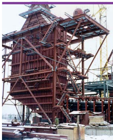
Installation of boiler P-92 for PO NAFTAN
