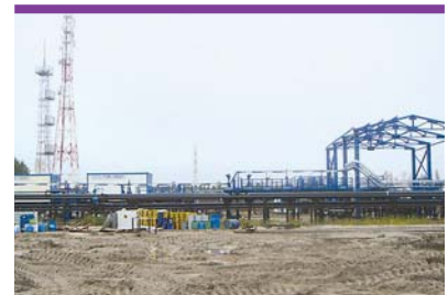
Construction and installation works. Urnskoye field
