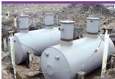
Deepening of underground tanks. Urnskoye field
